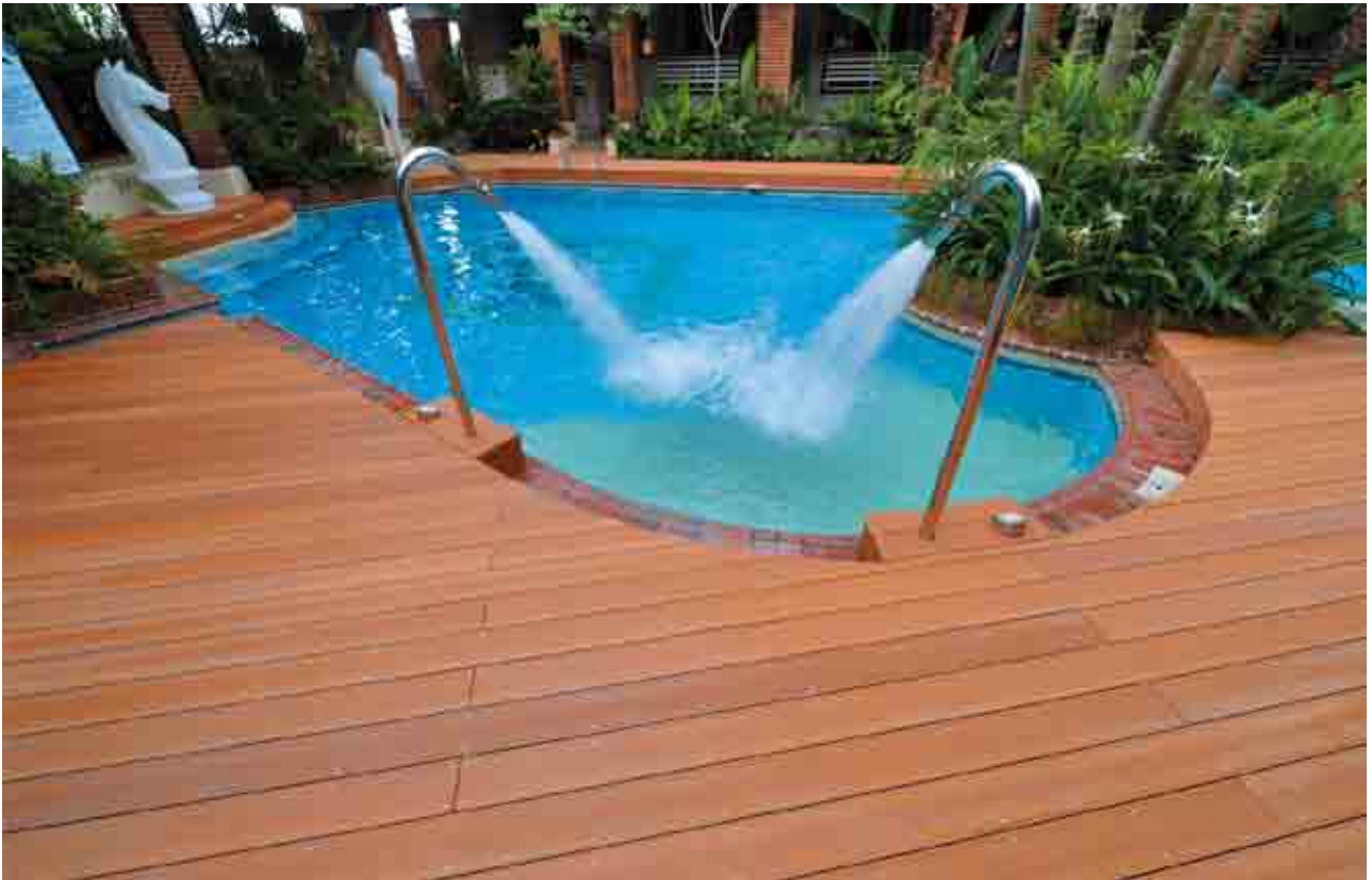
Outdoor Swimming Pool Decking 戶外泳池畔用地板
