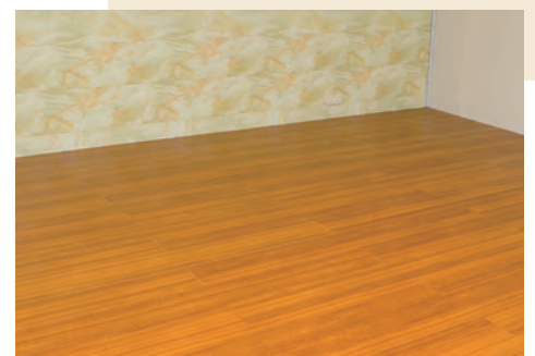
舒活地板施工完成 Completion of the ECO flooring tile construction
